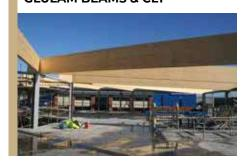
Glulam beams are a lightweight, eco-friendly alternative to concrete and steel beams providing an attractive natural look for large open spaces. Our large range of Glulam sizes can be used for a wide variety of applications including straight, angled and curved frameworks.
